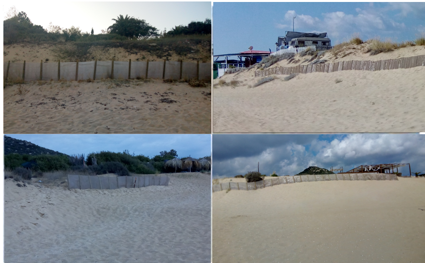
Figure 2. Sand fences for coastal restoration installed in Ammolofi, Greece.
