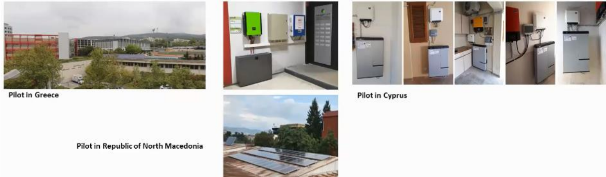
Figure 4: Indicative images of the PV ESTIA project
