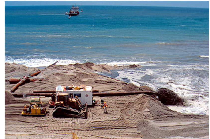
Beach nourishment works
